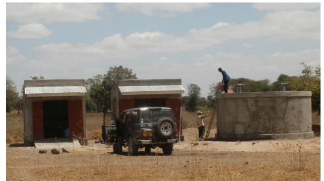
Phase 1 Completed Supply Generator, Pump and Water Tank
