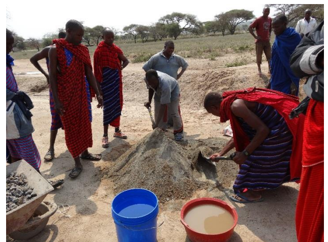
Phase 2 Village Participation digging and laying pipeline
